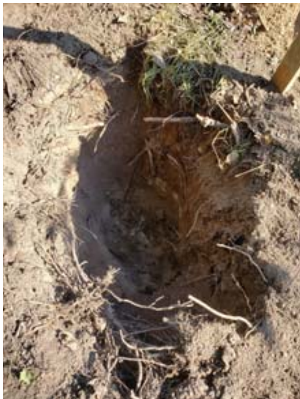
Large postholes are needed for sturdy fence post installation.
